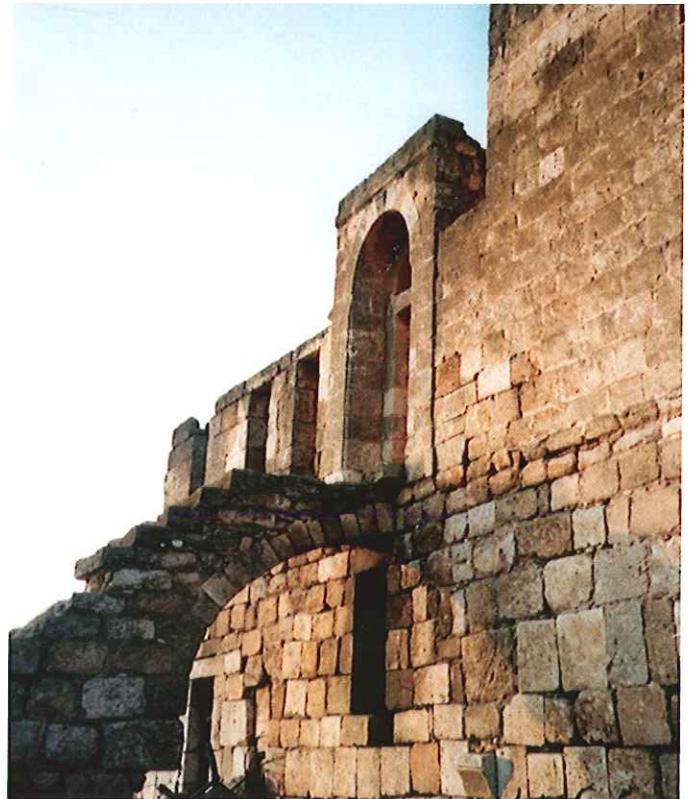
North façade of the Qasr, facing southwest. Note the construction of a second story, an external staircase, and beams, which would have supported a balcony. Photo courtesy of Lynda Carroll.
