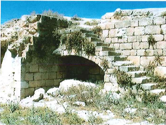
Remains of storage rooms and a central courtyard, with a staircase leading to the roof of the structure. The road (left), which leads into the modern village of Hisban, was constructed in the 1970s, bisecting the structure. Photo courtesy of Lynda Carroll.
