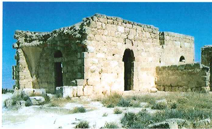
Second story of the Qasr. When in use, the upper story contained at least three rooms with dome-vaulted ceilings and was accessed by an external staircase. Photo courtesy of Lynda Carroll.
